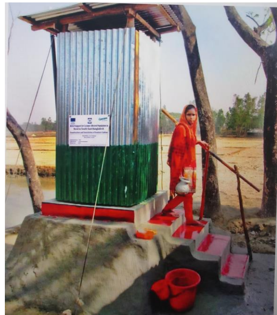
Figure 5: Elevated latrine, Satkhira, 2021
