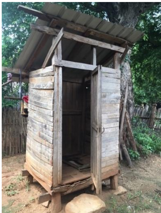
Figure 7 and 8: Examples of elevated off-set pit latrines in a village in rural Nyaung U, Myanmar
