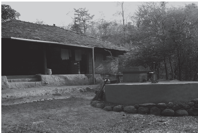
Individual rooftop rainwater-harvesting structure: People help themselves (Source: WASMO)
