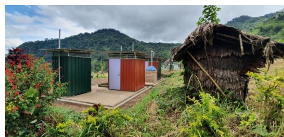
Photo 1: Climate resilient school latrines in Papua New Guinea
