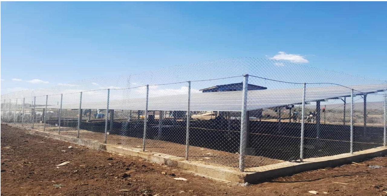
Figure 8: Solar array constituted of 162 solar PV panels powering the Hariro water supply system. (@UNICEF Ethiopia/2023)
