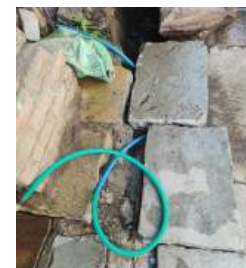
FHTC Pipe run through the drainage in Pandmodi Village
