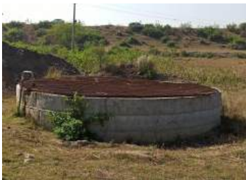
Fig: Capped openwell of Gadola
