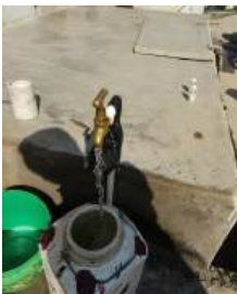
FHTCs are placed at the entrance (Panmodi Village)
