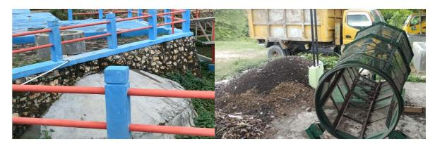
The biodigester in the IPLT Gempong Jawa (Banda Aceh) generates gas that can be used as a source of energy (left picture) and the sieving facility used at the IPLT Koya Koso (Jayapura) produces finer sludge particles to be used as a soil enrichment material (right picture).
