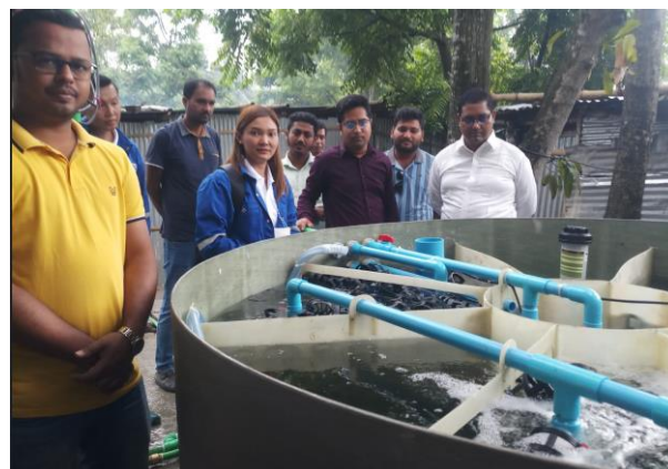
Figure 7. Testing of the SBR wastewater treatment system at a low-income settlement of Rajshahi City
