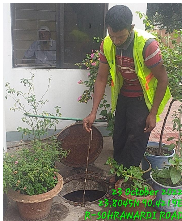
Figure 4. DNCC staff carrying out compliance assessment of a containment system in a DNCC ward
