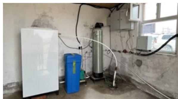
Figure 6: Water purification filter at the smart water kiosk in Jargalan sub-province, Gobi-Altai
