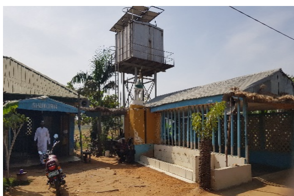
Figure 6: Public latrine along Hadejia major road for travelers
