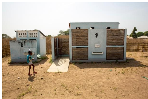
Figure 2. A student walks past a newly constructed school latrine block with a ramp in Sintchan-Farba, Guinea-Bissau
