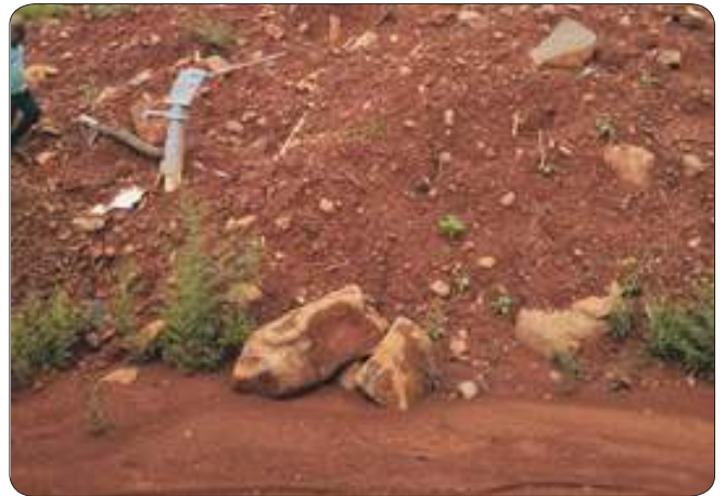
Handpump reinstated after landslide in Posare Village, Khed Taluka, Ratnagiri District
