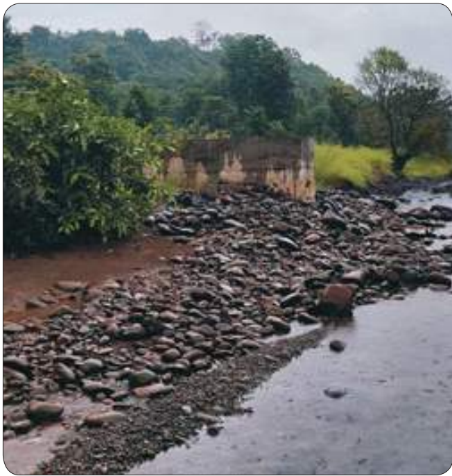
Construction of new well in Posare Village, Khed Taluka, Ratnagiri District
