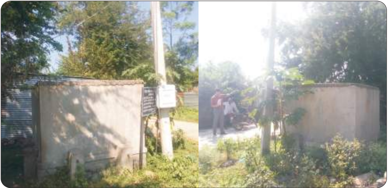
Field Visit in Nandurga Village, Ausa Block, Latur District, Exploring the reasons for the failure of the borewell based scheme
