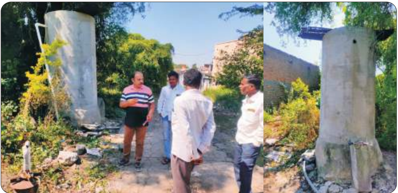
Field Visit in Pangaon Village, Renapur Block, Latur District, Understanding the root cause for the failure of the borewell based scheme
