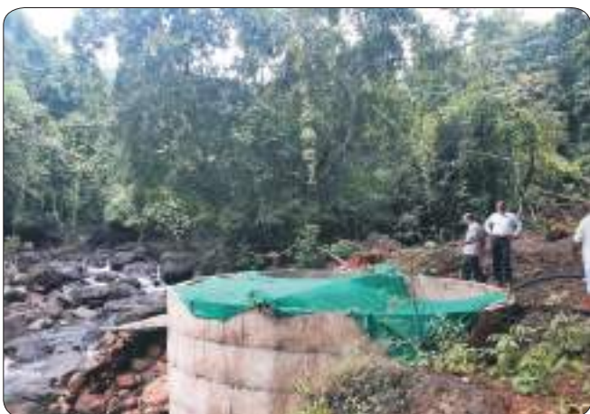
Covering the well to protect it from plant debris in Aare Village, Guhagarh Taluka, Ratnagiri District
