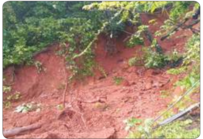
Well filled with landslide debris in Vetoshi village, Ratnagiri Taluka, Ratnagiri District
