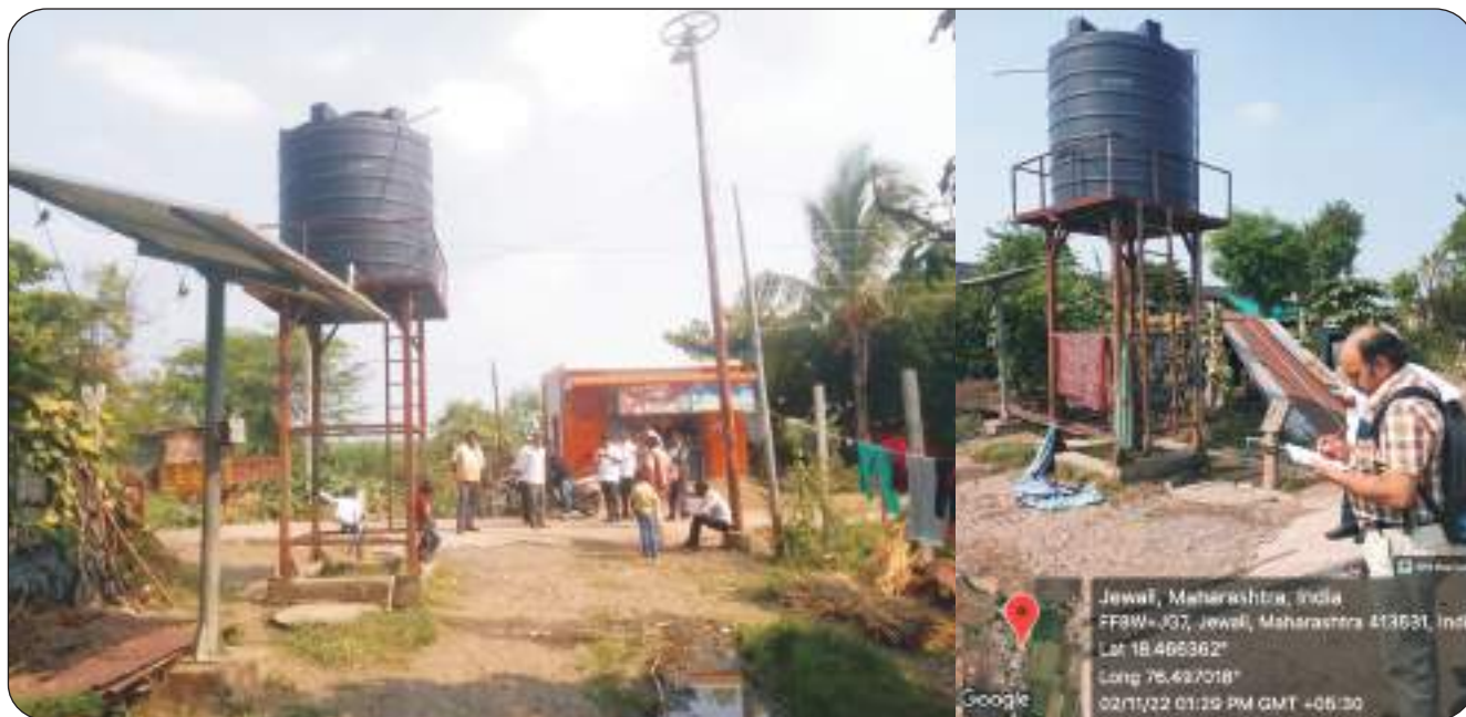
Field visit in Jewali Village, Latur Block, Latur District: studying the failed bore wells
