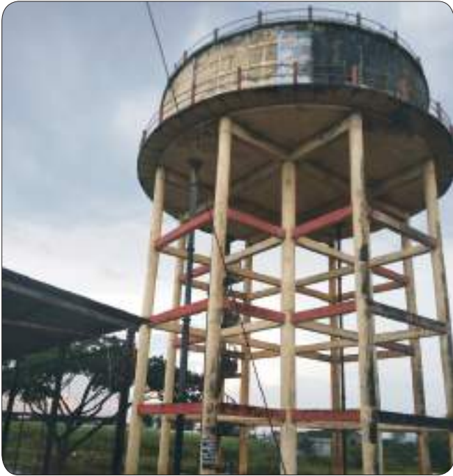
Water reservoir structure in Kolhapur
