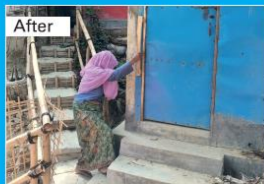
Figure 5: Sholema approaching upgraded latrine.
