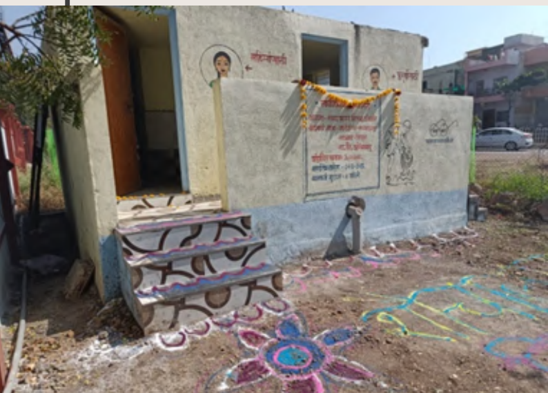
A PUBLIC TOILET IN THE GP
