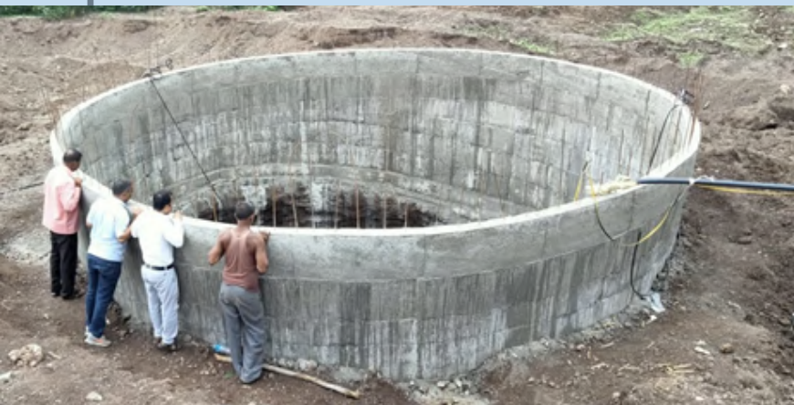
CONSTRUCTION WORK OF SOURCE WELL
