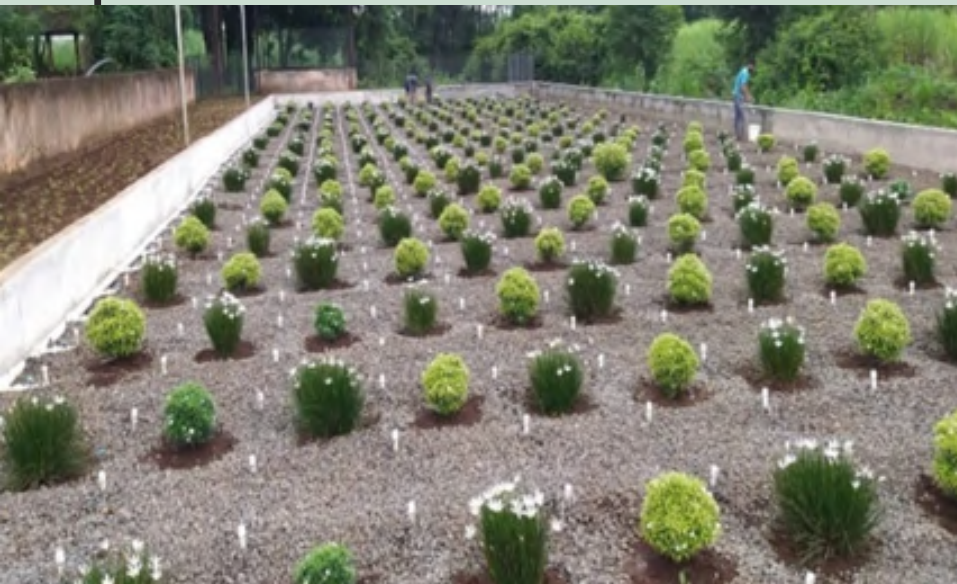
STP AT KUNDAL GP
