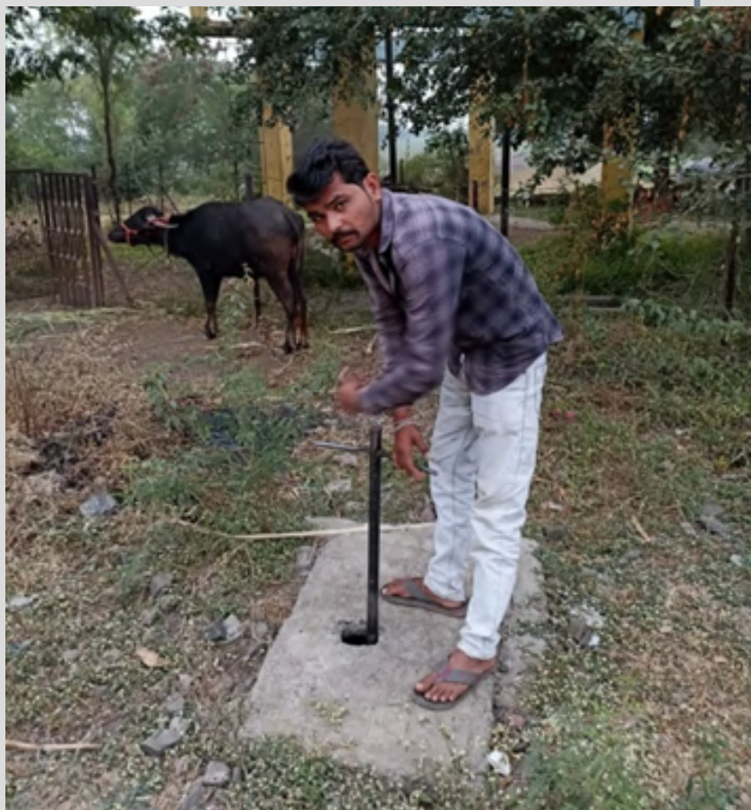
WATER PERSON OPERATING THE VALVE FOR WATER SUPPLY
