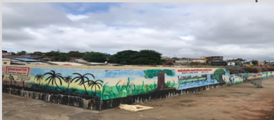
STP (CAPACITY 1 MLD)
