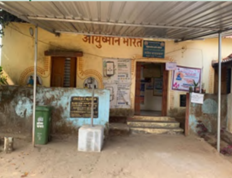
INSTALLED COMMUNITY LEVEL BINS
