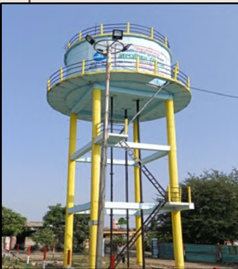
WATER STORAGE TANK
