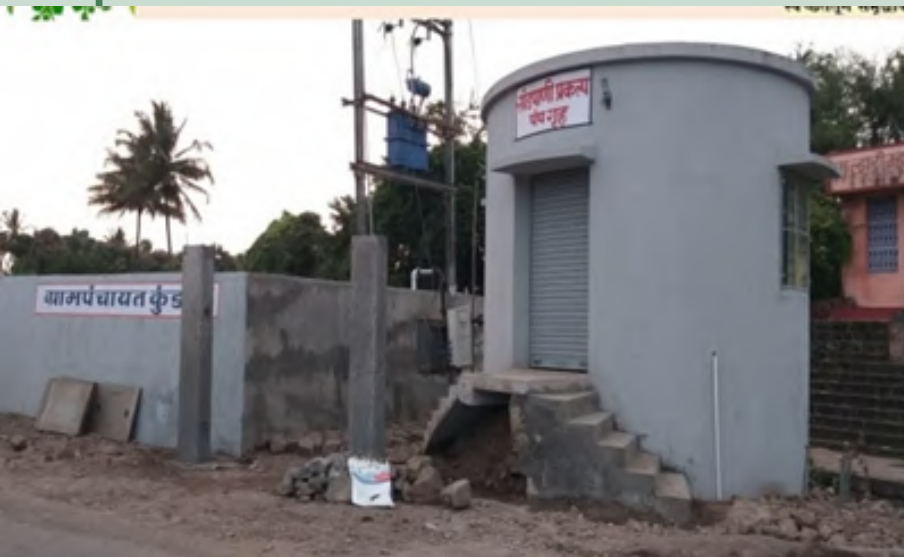
PUMP-HOUSE NEAR STP
