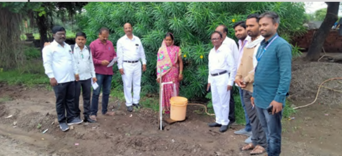
SURVEY OF FHTC INSTALLED AT A HOUSEHOLD
