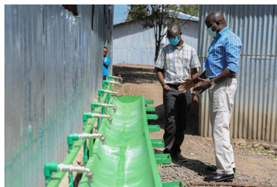
Figure 4. UNICEF WASH Chief at Ethiopia, tests the metal pedals of the hands-free hand-washing stand designed by Steven Mugarra, UNICEF WASH engineer
