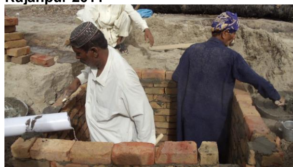
Figure 4: Construction of elevated latrine, Rajanpur 2011
